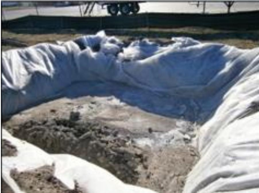
Plate 3-2 Concrete Washout Area
