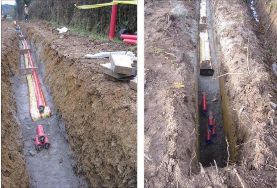
Plate 2-1 Typical Cable Trench View
