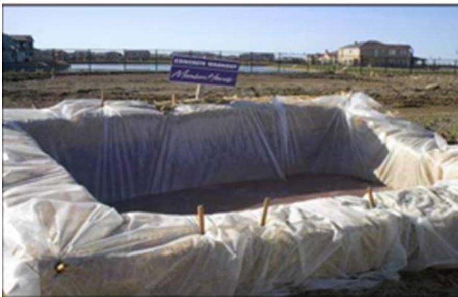
Plate 3-1 Concrete Washout Area
